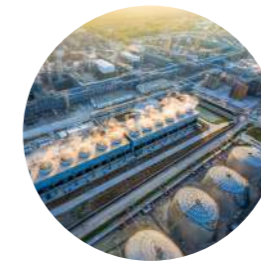
Chemicals for open & closed cooling systems
