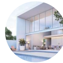
Whole-house water treatment
