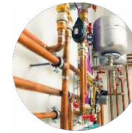
Heating systems filling
